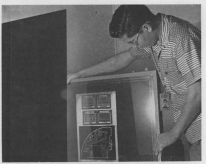
"BURNING IN" the image onto a sheet of pre-sensitized copper clad laminate is Dick Chavez. The process takes about four minutes under a high intensity arc-lamp to obtain a good pattern fix.
